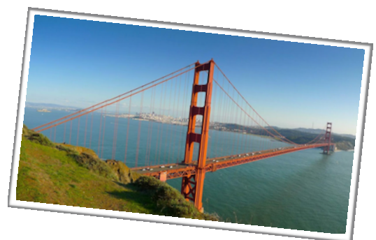
The Golden Gate Bridge (San Fransisco)
